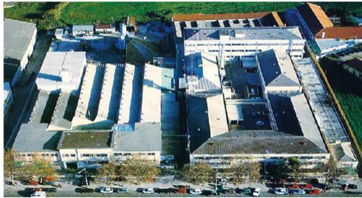
Lisbon (Portugal) Water meters
