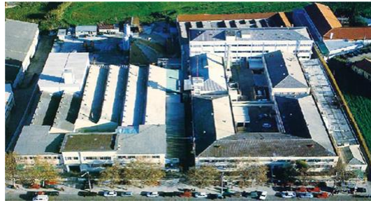
Lisbon (Portugal) Water meters
