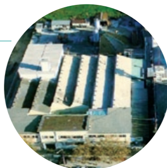
Lisbon (Portugal) Water meters
