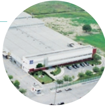
Monterrey (Mexico) Mechanical controls, sensors
